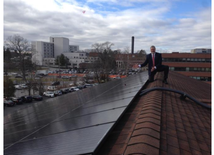
Executive Director Brian Skanes shows off the Club's commercial installation of solar panels.
