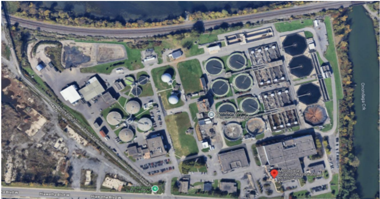
Metropolitan Syracuse Wastewater Treatment Plant.
