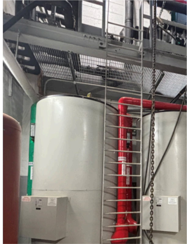
New high-efficiency, gas-condensing boilers and hot water tanks were installed for the projects at Jackson Houses and Eastchester Gardens.
