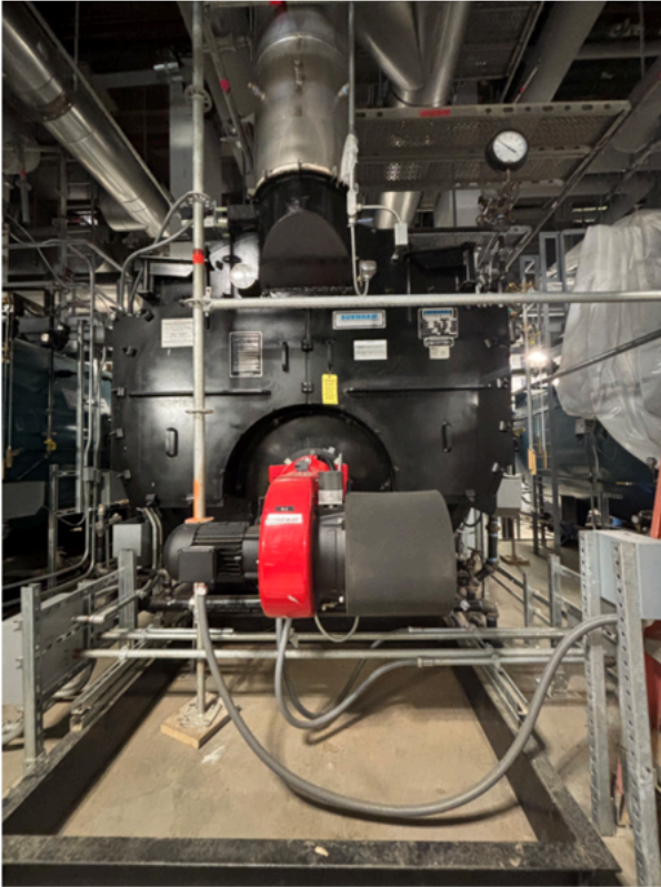
New high-efficiency, gas-condensing boilers and hot water tanks were installed for the projects at Jackson Houses and Eastchester Gardens.
